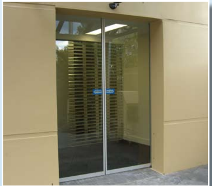
Designed for safer disabled access.
